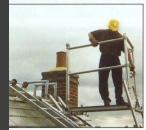
Fit handrail and engage interlock clips.
