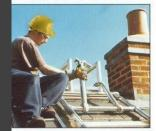
Secure the frame to the ridge unit with the ridge frame connector.
