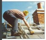
Fit single width frame to ridge unit by offering the spigots up to the ridge unit sockets, engage interlock clips.
