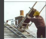
Position the platform on the appropriate rung of the frame.
