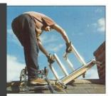
Place ridge unit over the ridge of the roof. Ensure that the wooden bearers are placed flat against the roof tiles.
